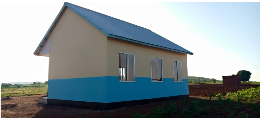
Pre-primary Infrastructure improvement support
